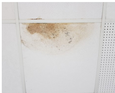
Figure 1: This picture shows the cellulose ceiling board in procedure room 6B. It was stained brownish by watermark, and the black-green patches were foci of fungal growth. The ceiling board was eventually replaced during rectification process.
